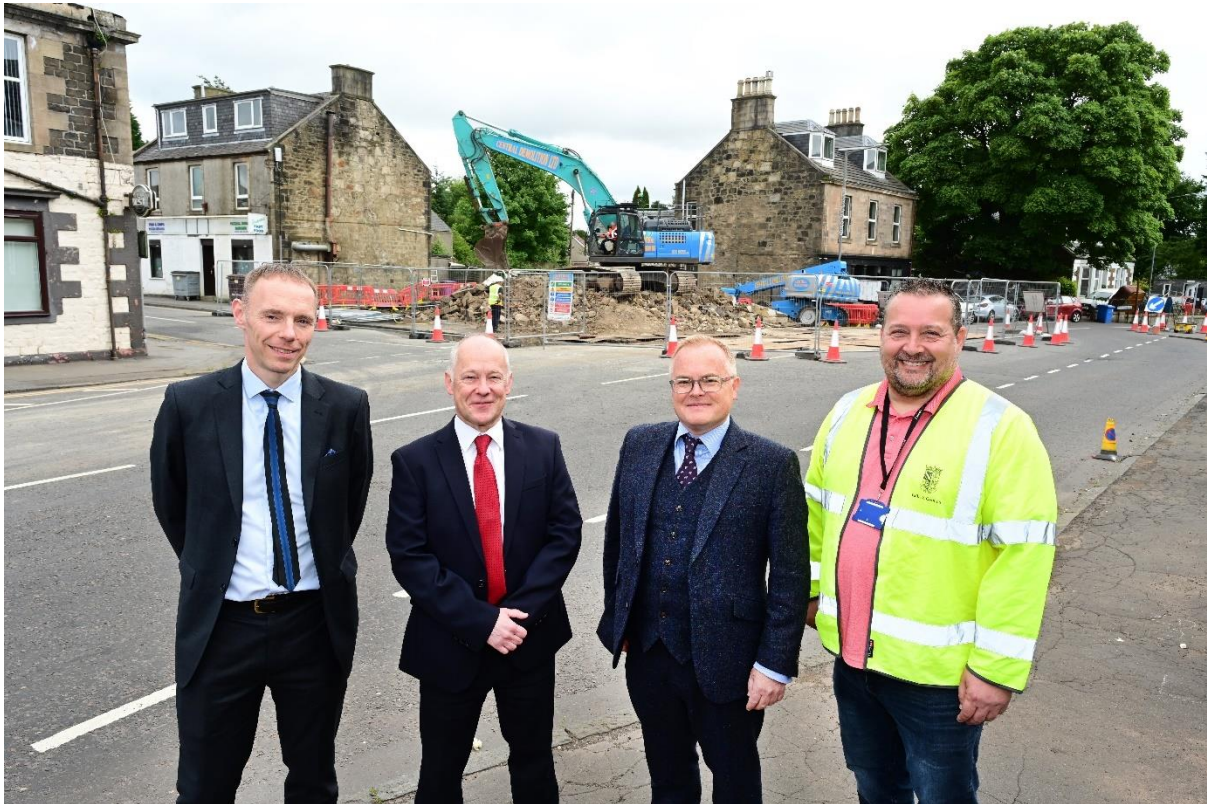
Demolition of former site of the Slamannan Hotel
